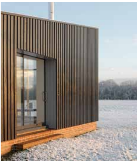
Exterior board on board timber cladding.
